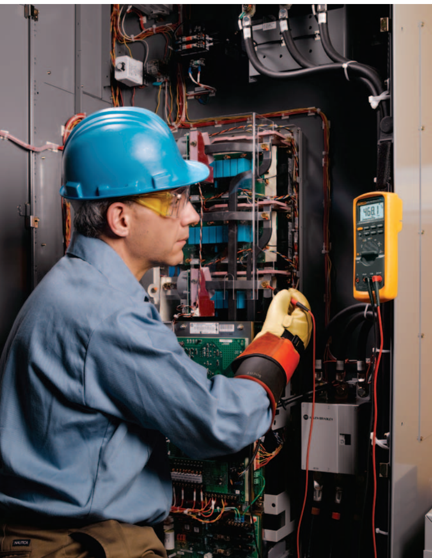
Thanks to its selectable low pass filter, the Fluke 87V DMM can accurately measure adjustable speed motor drives.
